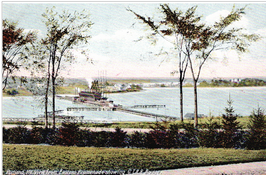
An impressive wooden viaduct with a steel swing span was constructed to bridge Back Cove in Portland and India Street on the Portland peninsula.
