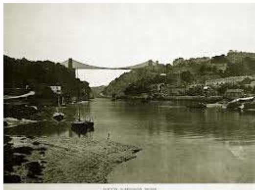
Fig.1 Brunel's suspension bridge at Clifton – completed 1864
