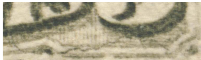
Figure 2. The major crack at lower right, in closeup.
