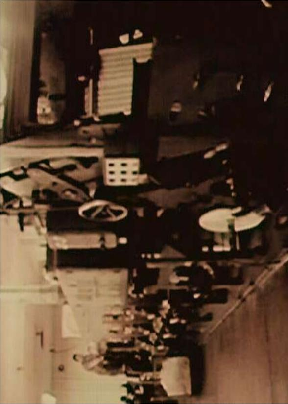
Figure 11. Like Figure 8, side view of the Goebel press but from the opposite end with the intaglio unit in the foreground. [Source: *Something Canadian*]
