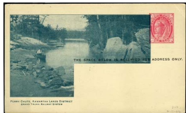
Fig. 2: GTR Column B, with framed view.
