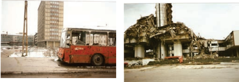
Figure 4. Mortar destruction, Sarajevo 1995.
