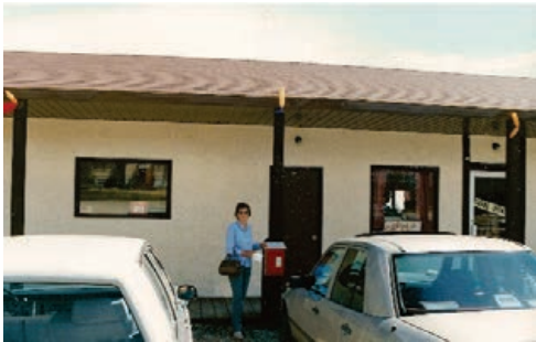
Figure 5. Waterford Valley Post Office 1989.
