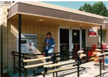
Figure 6. Okotoks post office built in 1969, photographed in 1988. The late Betty Speirs (the author's mother) is seen posting some covers. One of the covers was returned to her with the machine cancel shown in Figure 7.
