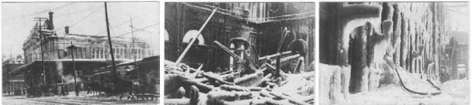
Figure 6. Pictures showing the aftermath of the fire of 1916.
