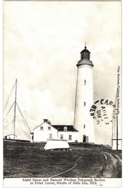
Figure 15. Wireless telegraph station at Point Amour, Labrador.
