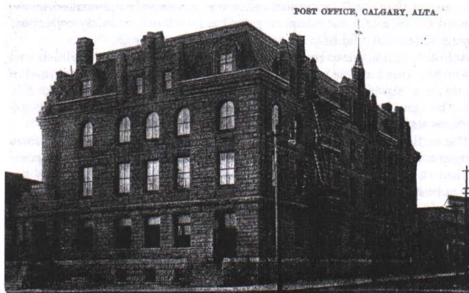
Figure 2. Second version of Calgary post office (1908–1914) Showing the fourth full storey.
