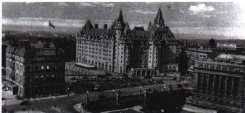
Figure 32. Rear of Ottawa post office
