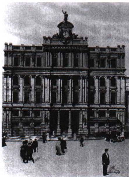
Figure 16. Architectural drawing of the Montreal post office The completed building had a different roof line, and no statue above the clock.
