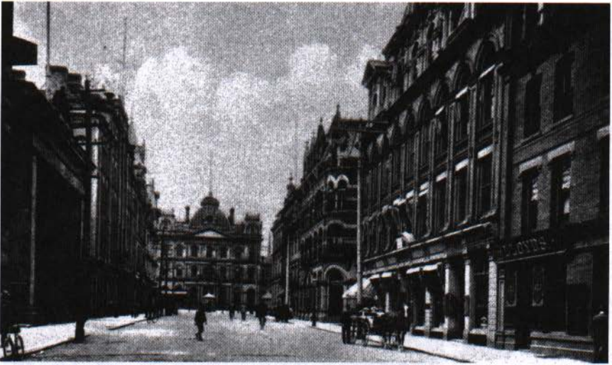
Figure 14. Second Empire post office in Toronto (completed 1874) Showing its location, which creates a grand formal prospect in the streetscape.
