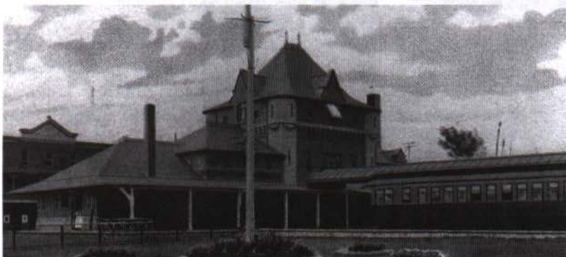
Figure 34. Rear of CPR Station, Ottawa
