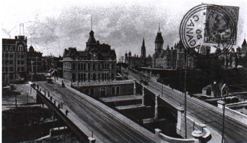
Figure 6. View of pre-1904 Ottawa post office On left is Sappers Bridge, at right, Dufferin Bridge. Post card is dated 1906.
