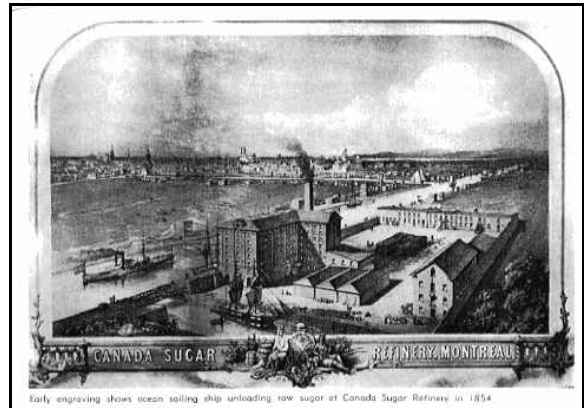
Aerial view of the Canada Sugar Refinery in 1854. (From the May 1867 issue of Industrial Canada .)
