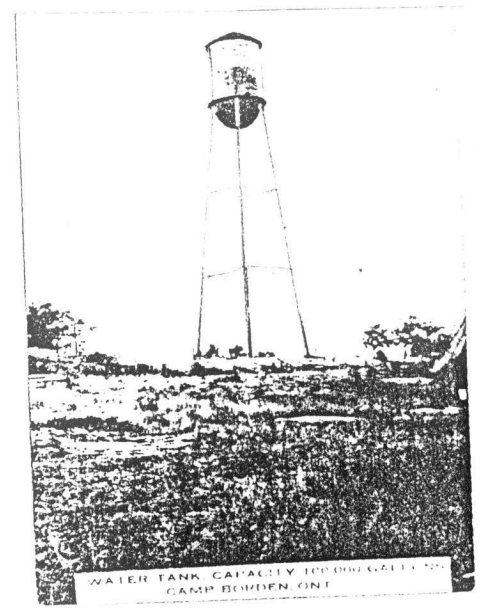
A FAMILIAR LANDMARK 100,000 GAL. WATER TANK
